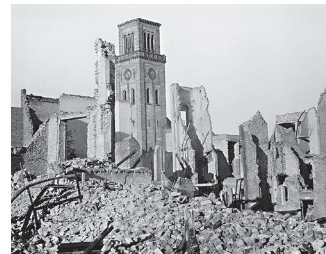
Fig. 11: St. Josef Church in Lindenhof in 1946, Viewed from Meerfeldstr. 11.
